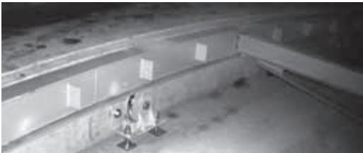
Fig. 13 Timber connection to peripheral beam arc HEA and places of wood prism elements attachment
