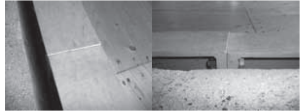
Fig. 6 Example of peripheral beam attachments of rotational airplane platform – view from above
